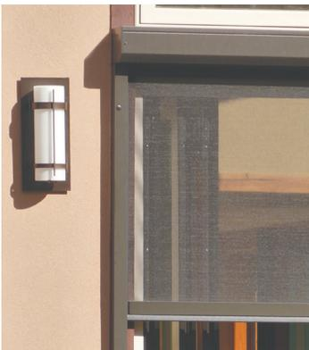
Face-mounted side tracks with matching plug buttons
