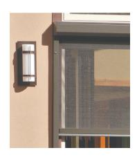
Face-mounted side tracks with matching plug buttons
