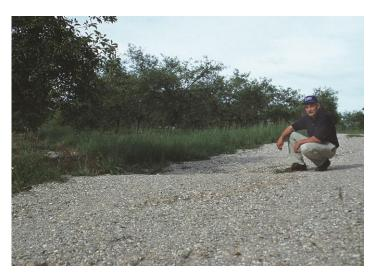
Figure D-4-1. "Resource Conservationist shows a water bar erosion control practice on a gravel road adjacent to an orchard. Grand Traverse County, Michigan." Source: USDA NRCS.
