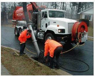
Figure D-10-1. Storm Drain Cleaning in Anne Arundel
