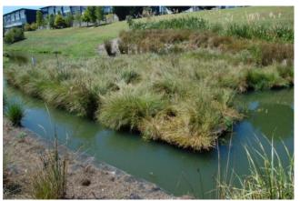
Figure D-11-1. A Floating Treatment Wetland (FTW) in an existing wet pond. Source: Bill Hunt, NCSU (see Expert Panel Report).
