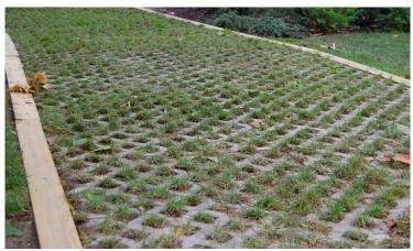
Figure D-1-2. Permeable pavement is a type of runoff reduction (RR) practice because it allows processes such as filtration and evapotranspiration to occur. This approach reduces runoff and removes a greater portion of pollutants than stormwater treatment (ST) practices that employ a permanent pool – such as wet ponds, wet swales, and constructed wetlands – because such practices simply provide storage and treatment before discharge. Photo: CBP.
