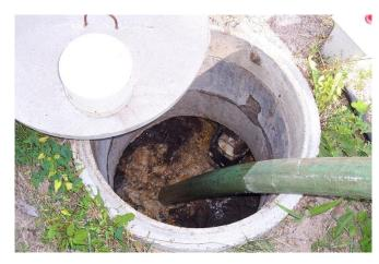
Figure S-1-1. Pumping sludge out of a septic tank, a routine part of septic system maintenance. Source: MCPA Flickr. (https://flic.kr/p/UScorM).
