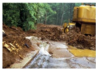
Figure D-3-1. Sediment running off a construction site. Source: Chesapeake Bay Program.
