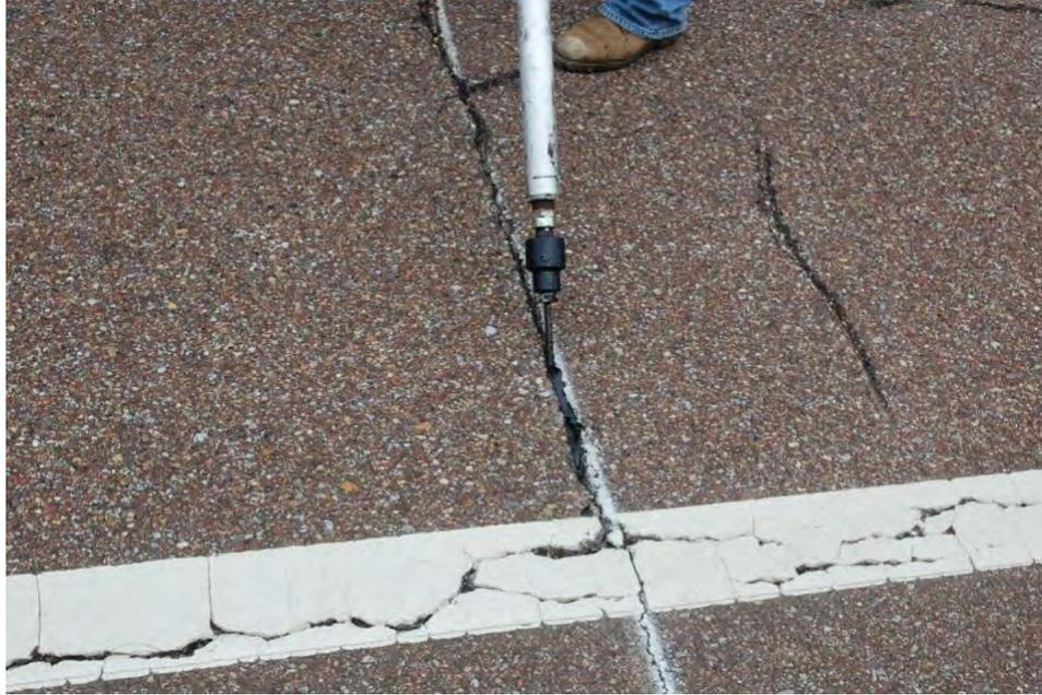
**Figure 4 Filling Cracks in Section S2A**
