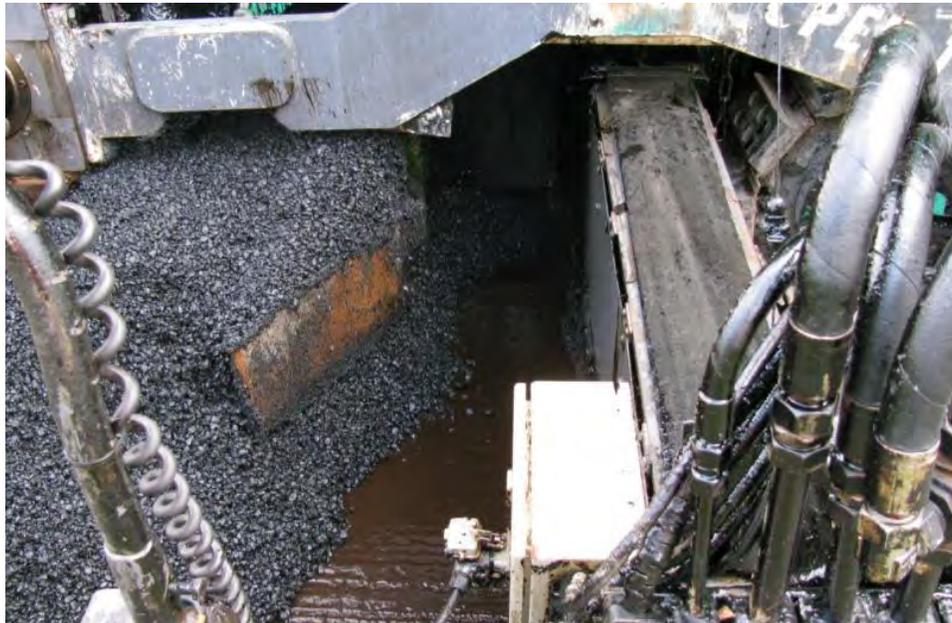
**Figure 1 Applying Thick Polymer-Modified Tack Coat Using Spray Paver**
