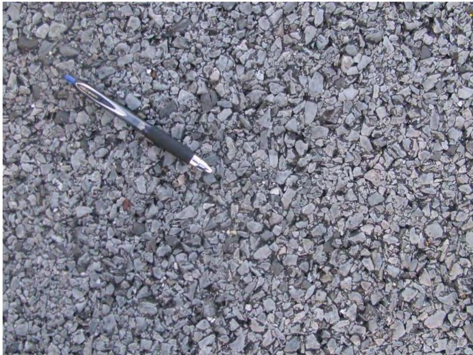
Figure 3 Section S4 Surface Appearance After 10 Million ESALs (2012 Cycle)
