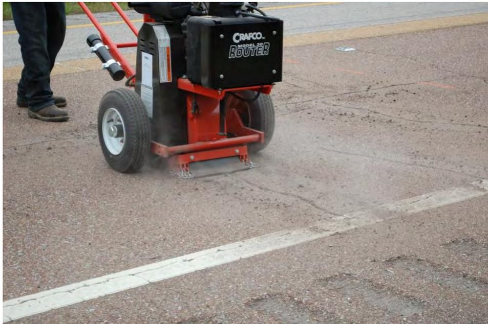
**Figure 3 Routing Cracks in Section S2A**
