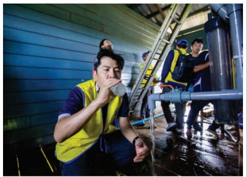
for a global grant from The Rotary Foundation. The grant allowed us to purchase the purification equipment and install it in five floating villages. The systems, developed by a Taiwanese company, can be reused for more than five years, and they work without electricity, which is not available in the floating villages.
