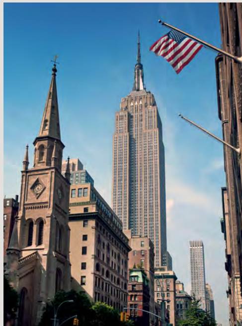
Empire State Building Shreve, Lamb, & Harmon - New York, NY - 1931
